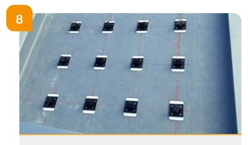
→ Overview of the roof once the pedestals are installed (There is no recommended orientation for the flanges of the pedestals in relation to the direction of the roof).
