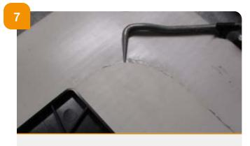
→ Once cooling, check the quality of the welds using the tester.
