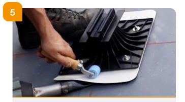
→ Welding on one side of the flange with a minimum width of 3 cm.
