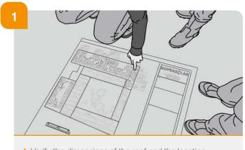
→ Verify the dimensions of the roof and the location of the hindrances in relation to the EXECUTION DRAWING before any marking.
