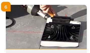
→ Weld the other side of the flange with a minimum width of 3 cm.
