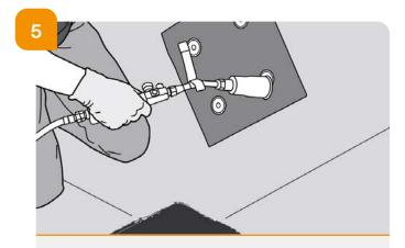
→ Heat up the flange using a propane torch.
