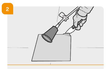
→ Heat up and remove the cutout section of the Aluminum finish sheet using the torch.
