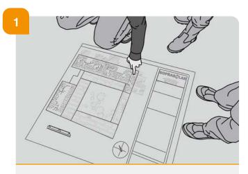
→ Verify the roof dimensions and the location of hindrances in relation to the EXECUTION DRAWING before any marking.
