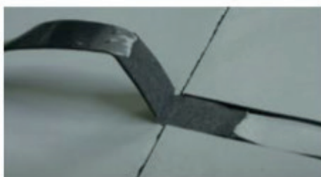
Pull from each side of the weld
